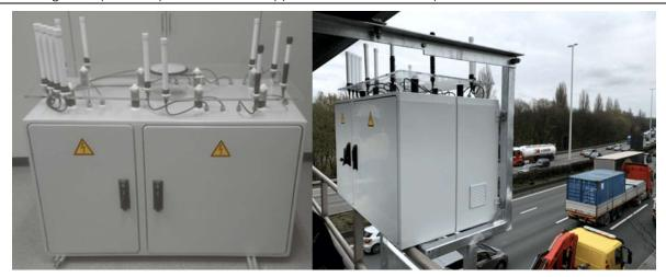
Figure 31: RSU on E313 highway
